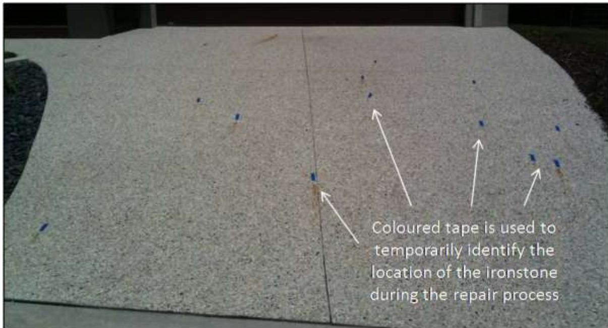
Start in one corner of the pavement, and methodically scan the surface, placing small pieces of the highly visible tape a few centimetres away from the epicentre of each identified Ironstone particle.
